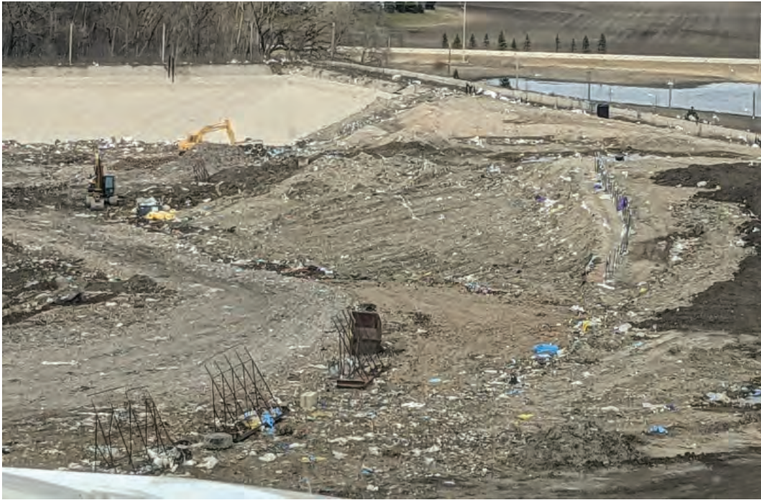
Phase 4, Northeast corner, well below crest
