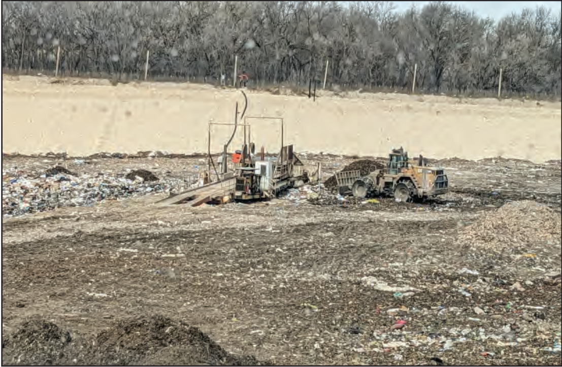
Tipper in Phase 4 at top of West slope
