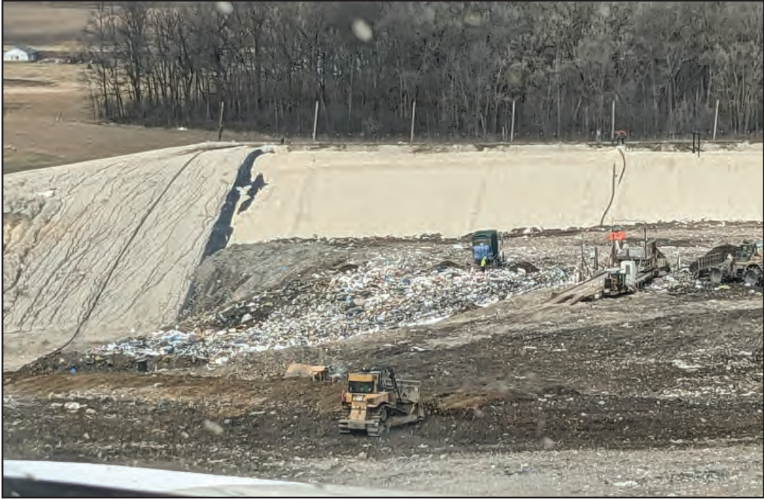
Tipping on West slope, outboard slope, finishing fluff layer
