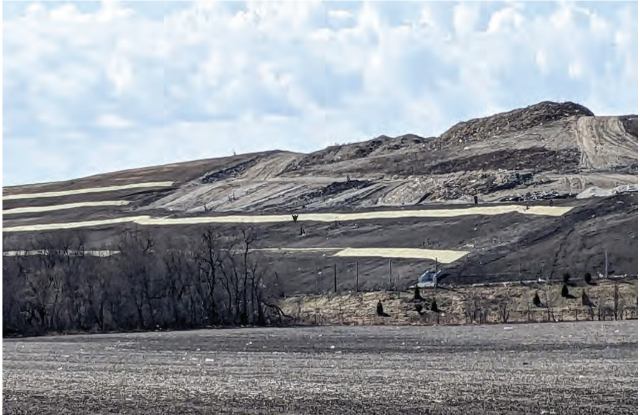
Capping project, East slopes
