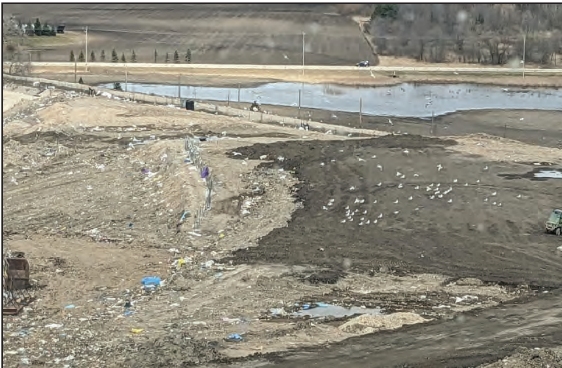
Phase 3 & 4 being brought to same elevation
