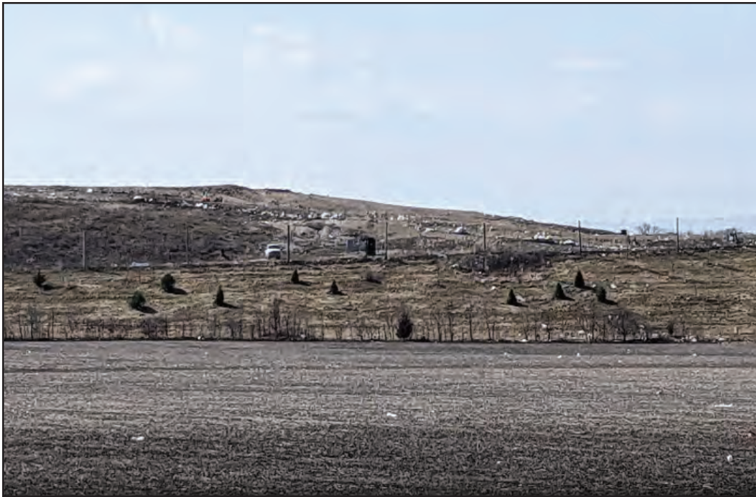
Northeast corner of Landfill footprint, high winds have spread litter
