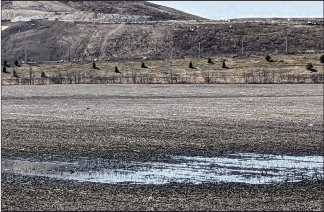
East slope of Phase 3 and 4 viewed from the Northeast
