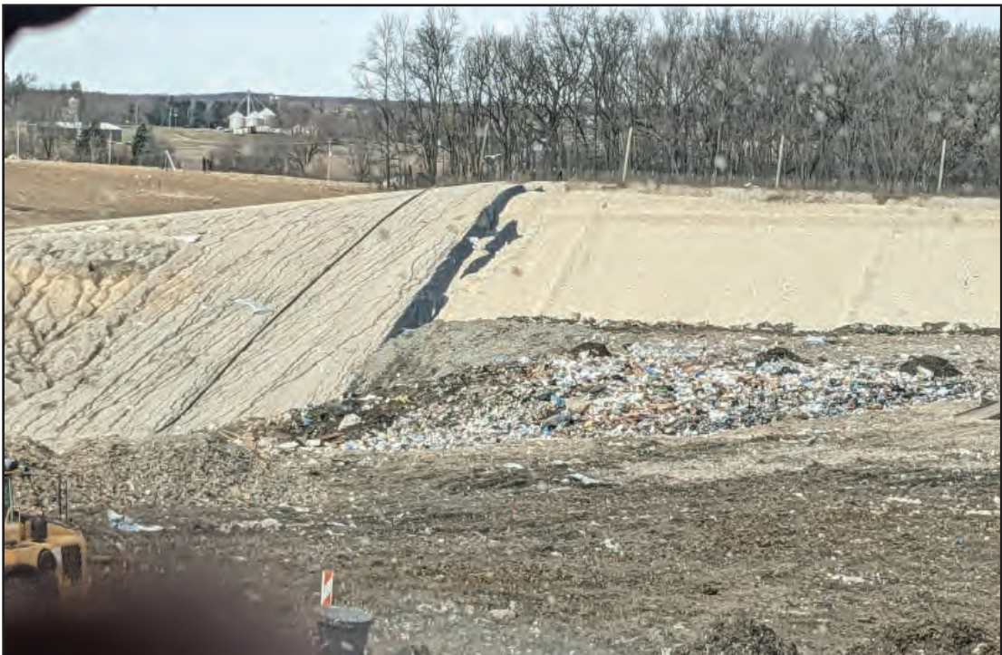
Tipping on West slope, finishing fluff layer
